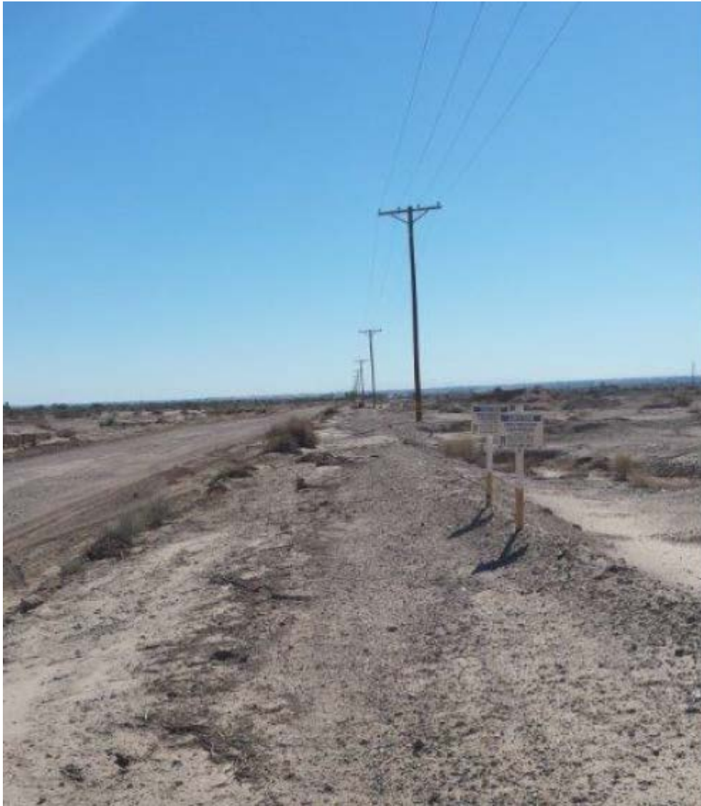
Figure 2.1. Existing electrical utility corridor with single-circuit pole assembly
