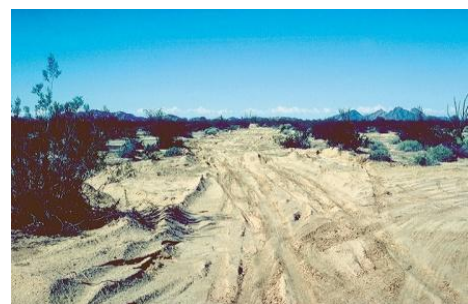
Inappropriate use and management of roads through the BMGR can result in accelerated erosion and affect surface flows.
